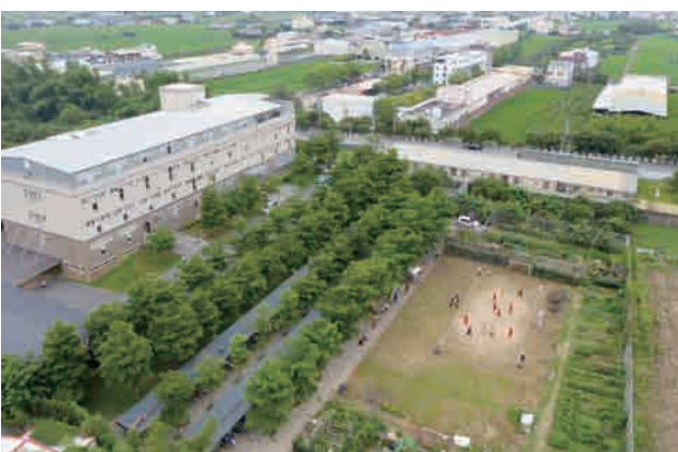
Migrant Workers' Dormitory
